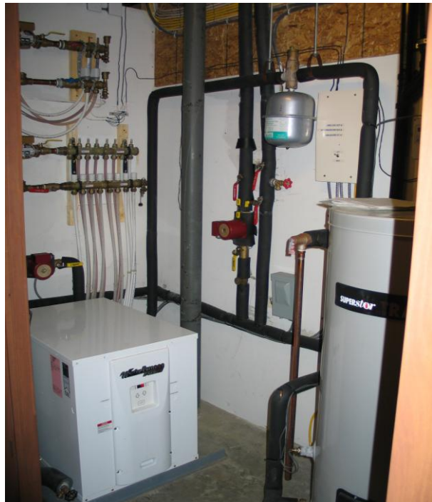
WaterFurnace EW series hydronic geothermal system for radiant heat with insulated stainless steel storage tank for heating and cooling.
