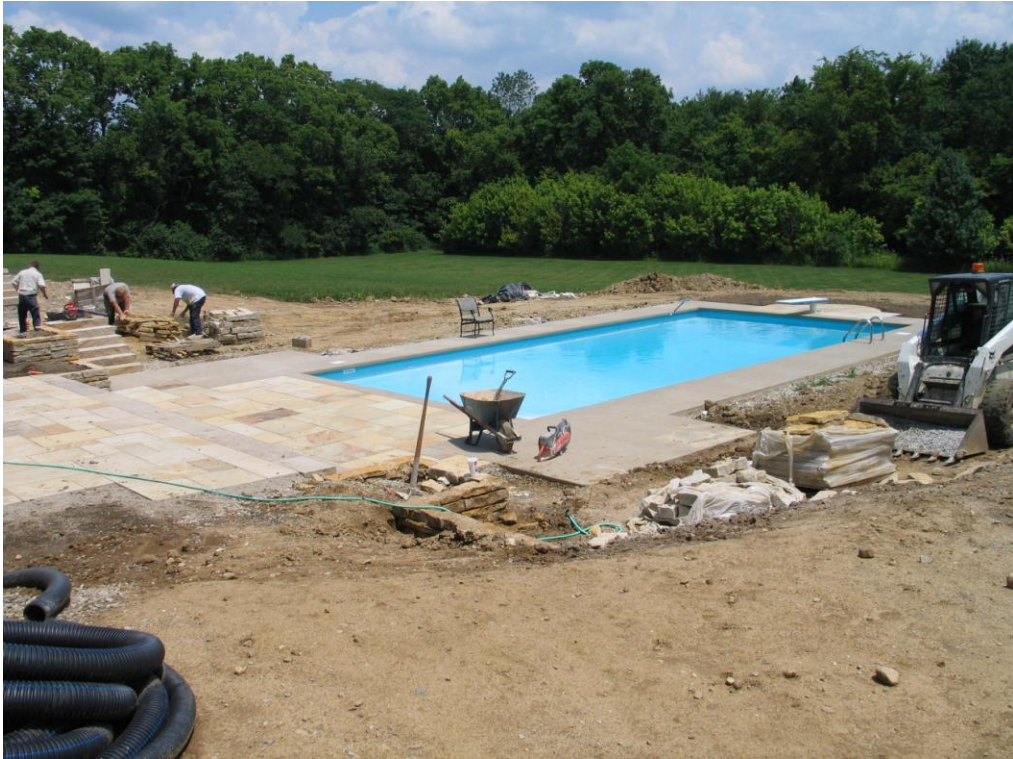
Pool under construction and ready for heating.
